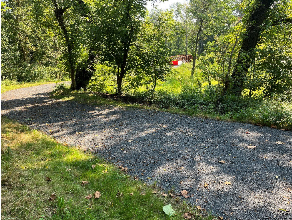
Figure 3 - Photograph from the vicinity of POD #1 looking southeast towards the Township trail. The existing berm can be seen beginning at the bend in the trail. Runoff that crosses the trail gets redirected by the berm and flows to the southwest towards the opening in the berm.
