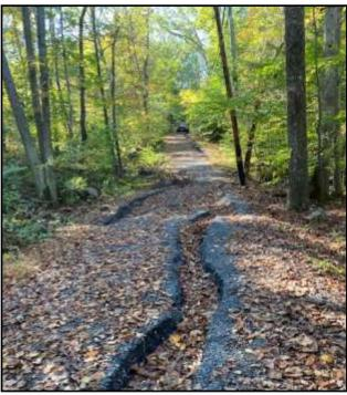
**BEFORE & AFTER:** King Rd in Salford Township received grant funding to repair a gravel road along the Ridge Valley creek that suffered severe damage during a large storm. The project including base repair, installation of a new culvert, and stone aggregate to improve the roadway and drainage. This project was started in 2021 and completed in 2022.
