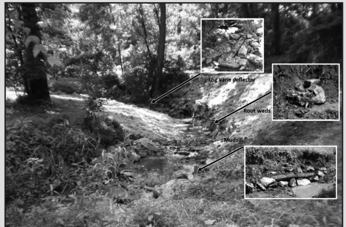
Perkiomen Creek post-construction: re-graded stream banks stabilized with seed and straw mulch after the structures were installed.
